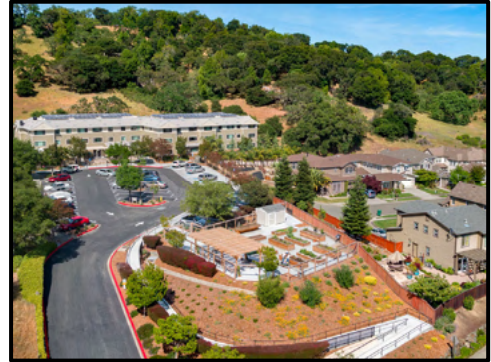
Mackey Terrace is located in Novato, CA. It is an affordable, special needs housing development that was sponsored by Eden Housing Inc., a nonprofit developer. It has 50 units with a density of 26 dwelling units per acre.
