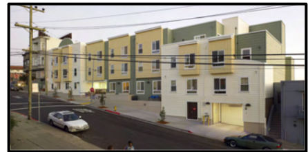
Hillcrest Gardens in Daly City, California is an affordable senior housing development with 40 units. It has a density of 100 dwelling units per acre.
