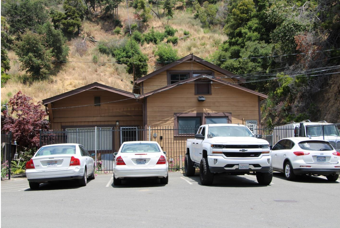
Primary Elevation of Maintenance Building, Camera Facing North.
