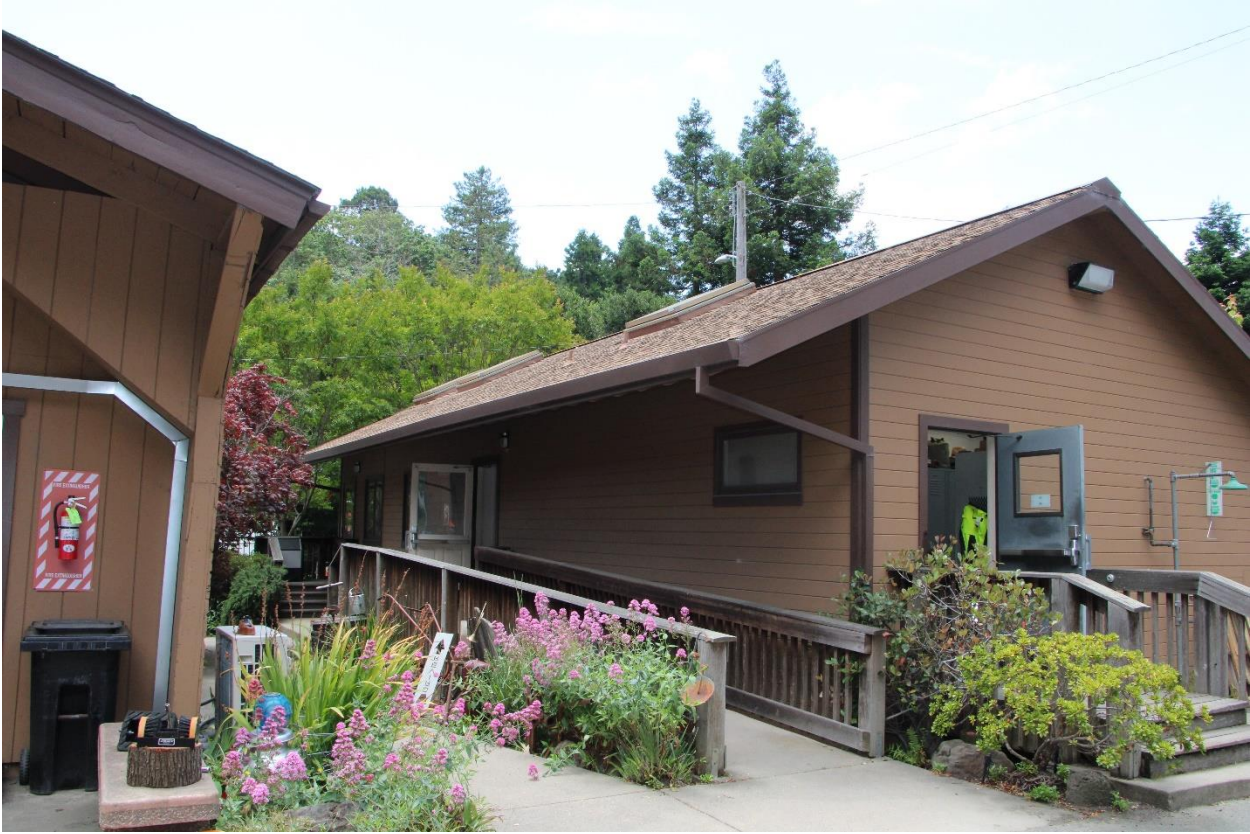
Figure 7 Rear and East Elevation of Office Building, Camera Facing Southwest
