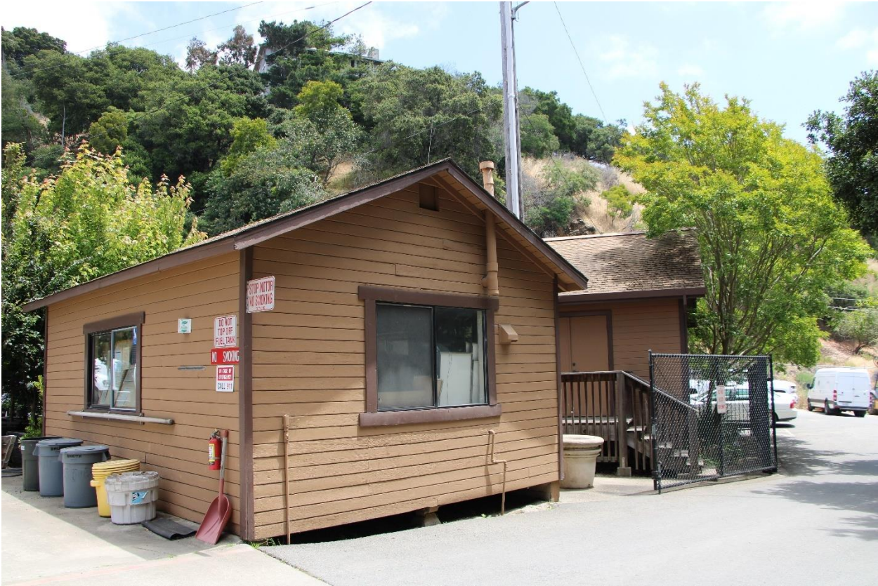
Figure 6 Primary and West Elevation of Shed Building, Camera Facing Northeast
