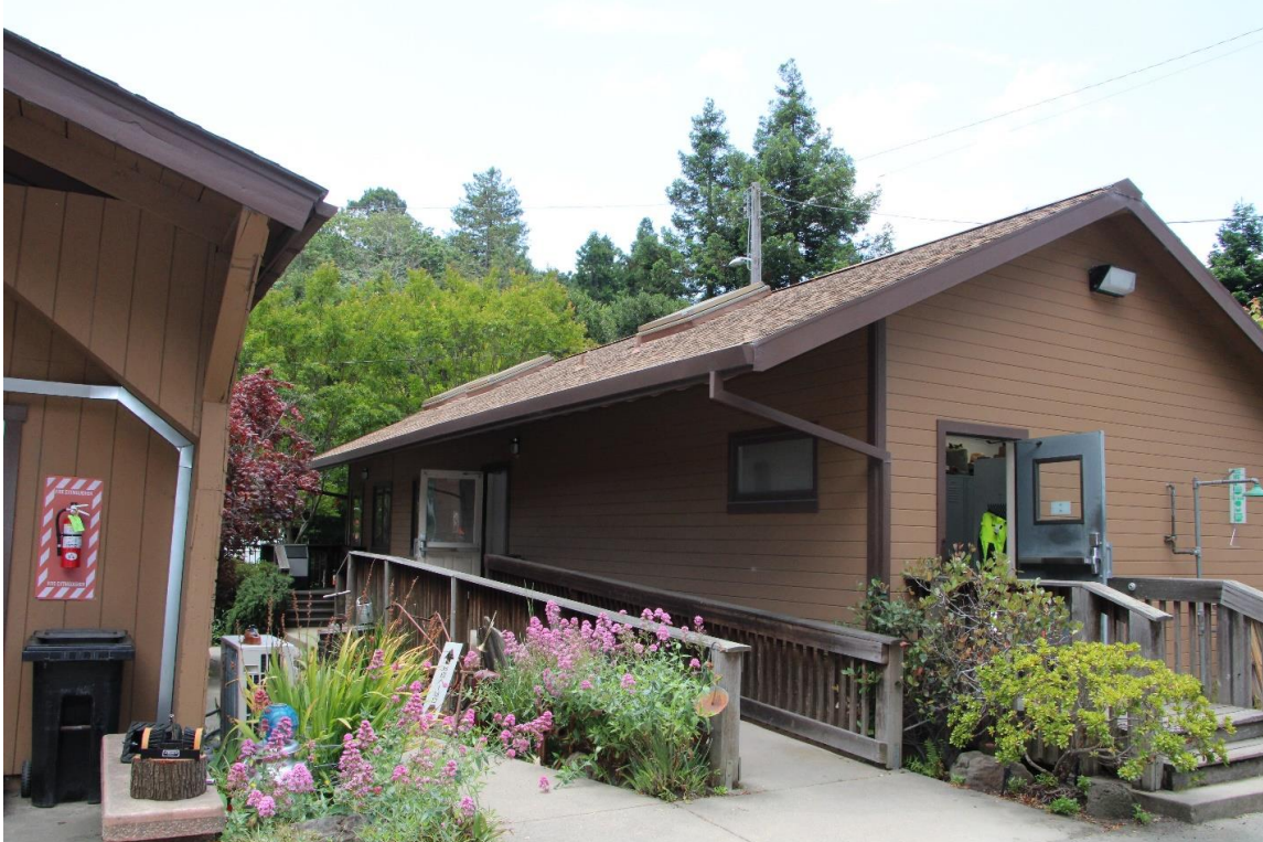
Rear and East Elevation of Office Building, Camera Facing Southwest.
