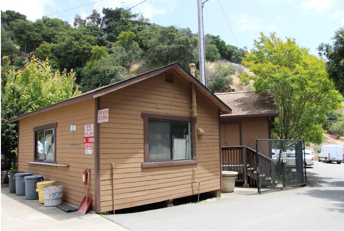
Primary and West Elevation of Shed Building, Camera Facing Northeast.
