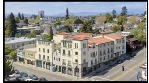
Il Piemonte in Oakland, CA, is a mixed-use development with all 26 units being market rate. This four-story development has a density of 89 du/ac.
